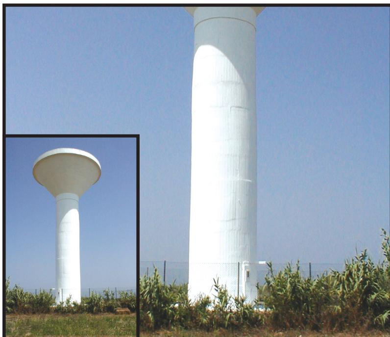
The concrete was suitably prepared to ensure that the substrate was clean, dry and free from contamination and primed prior to the application of our water-based, flexible coating Wall-Tech FP.
