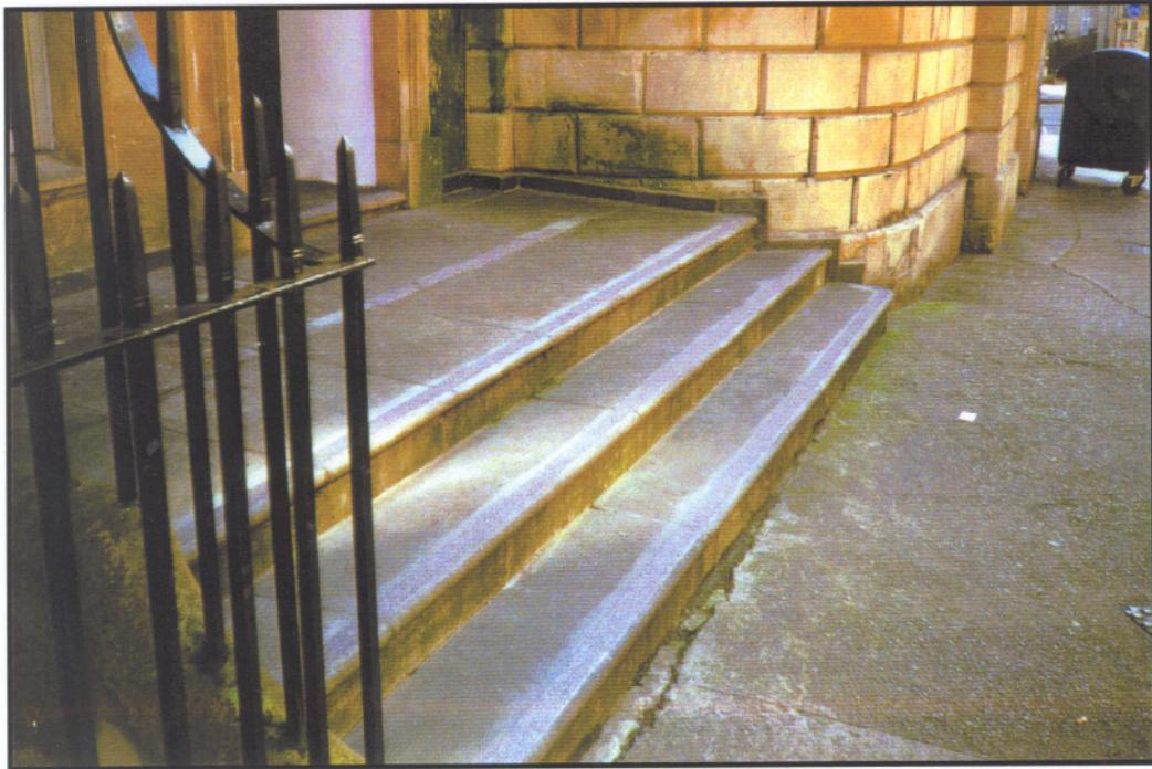
All dirt deposits and other contamination were removed from the concrete; the step nosings were then abraded. These abraded areas were then coated with Grip-Tech. This system is a solvent-free epoxy coating, which has been combined with an abrasion resistant aggregate. It has been specifically designed for use as a slip-deterrent safety system.
