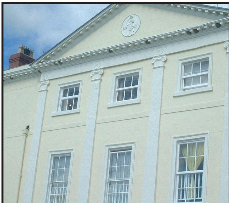
The façade of the building was cleaned and all loose and flaking material removed. Repairs to the concrete render were carried out using Wall-Tech LW, which is a lightweight concrete repair mortar, ideal for vertical and overhead surfaces.
